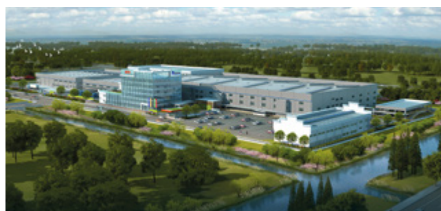
Construction of the new production platform in Nantong (China) is proceeding as scheduled.
